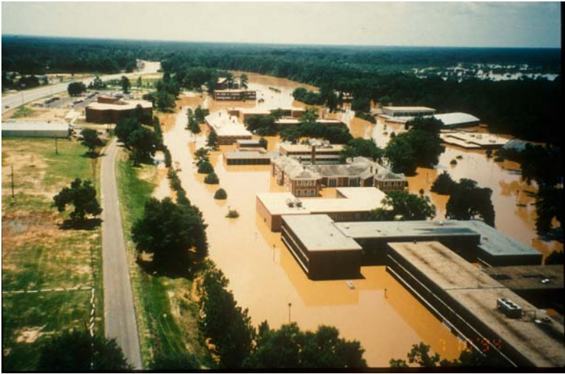
FIGURE 10. FLOODING INUNDATED THE ASU CAMPUS IN 1994.
