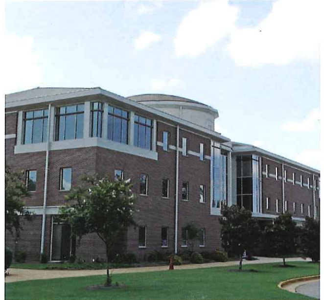
ACADEMIC SERVICES BUILDING: EXTERIOR
